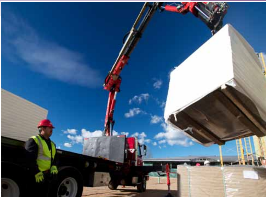
Below: Ricardo Alvaros of Allied Building Products, Denver, Colorado, operates the knuckleboom to unload commercial insulation on a new school construction job site in Boulder, Colorado. With speciality equipment such as this, Allied Building Products has the capability to deliver material directly to roofs up to 12 storeys high.
