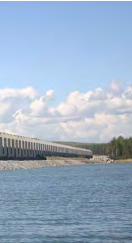
The Vuosaari Harbour project in Finland, to be completed in 2008, is one of Europe's largest harbour projects with 3.4km of new quay wall. Rudus delivered the concrete used in the construction of 675 high-quality quay elements at the site.
